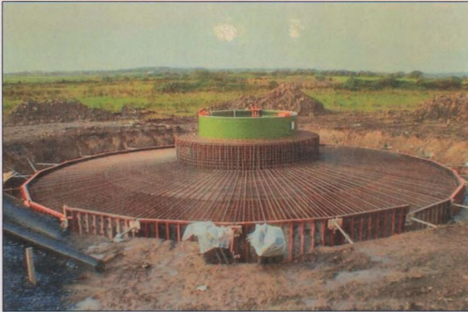
Plate 4-5 Image of Foundation at Ballywater Wind Farm taken during original Construction Phase
