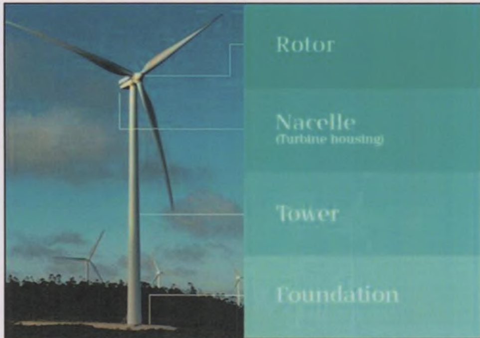
Plate 4-1 Wind Turbine Components
